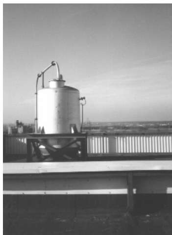
Rys. 2. Silos na granulaty polimerowe Fig. 2. Silo for polymer granulate
